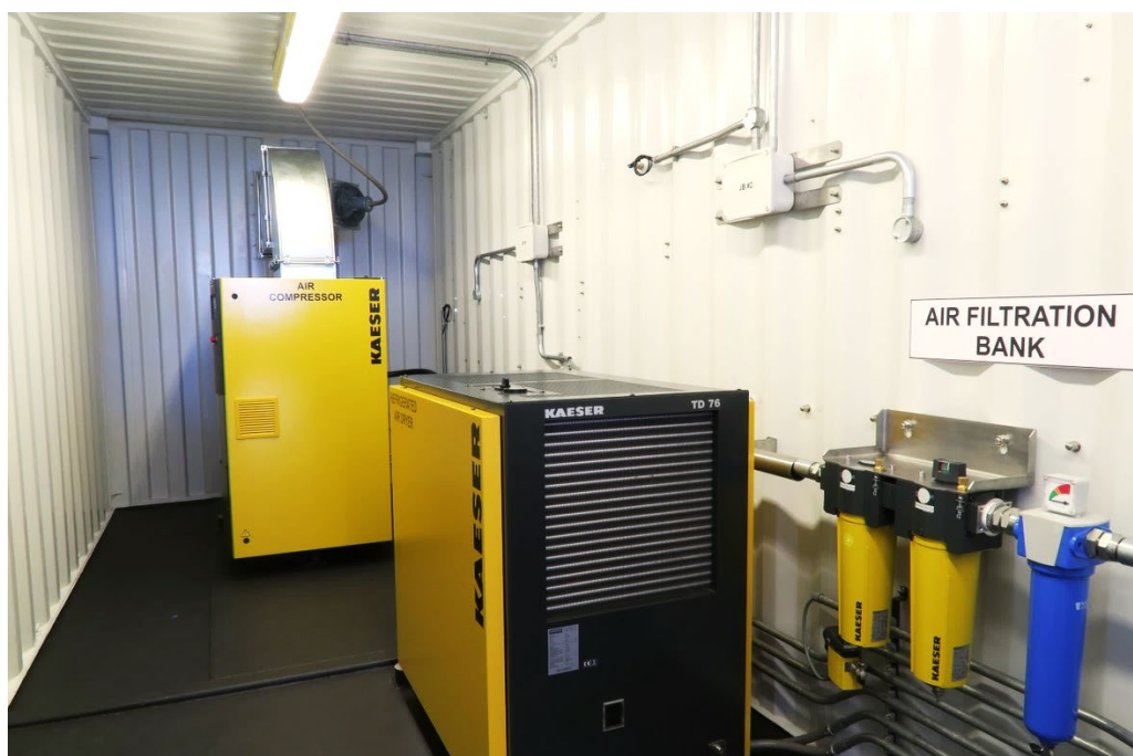
IMAGE 10: INDFOX-300-CT TYPICAL AIR SUPPLY EQUIPMENT
