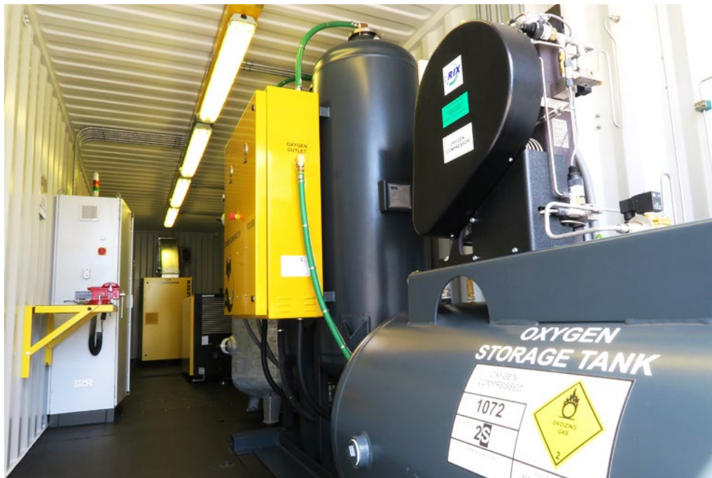
IMAGE 10: INDFOX-300-CT TYPICAL AIR SUPPLY EQUIPMENT
