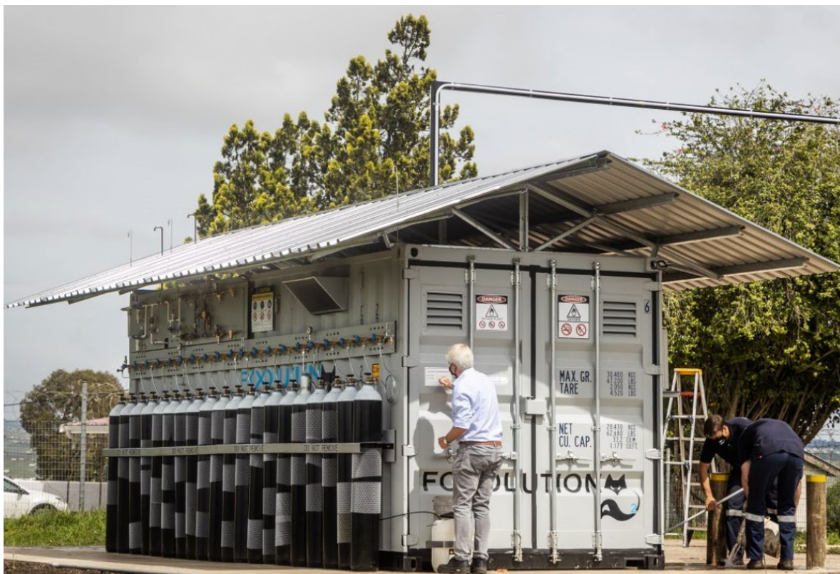
IMAGE 06: MEDFOX 10 -185-CT-DS CONTAINERISED OXYGEN 93% CYLINDER FILLING SYSTEM EXTERIOR
