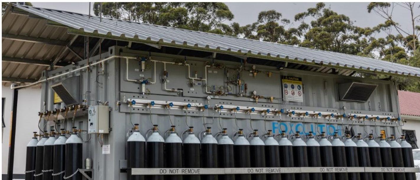
IMAGE 06: MEDFOX-185-CT-DS CONTAINERISED OXYGEN 93% CYLINDER FILLING SYSTEM EXTERIOR
