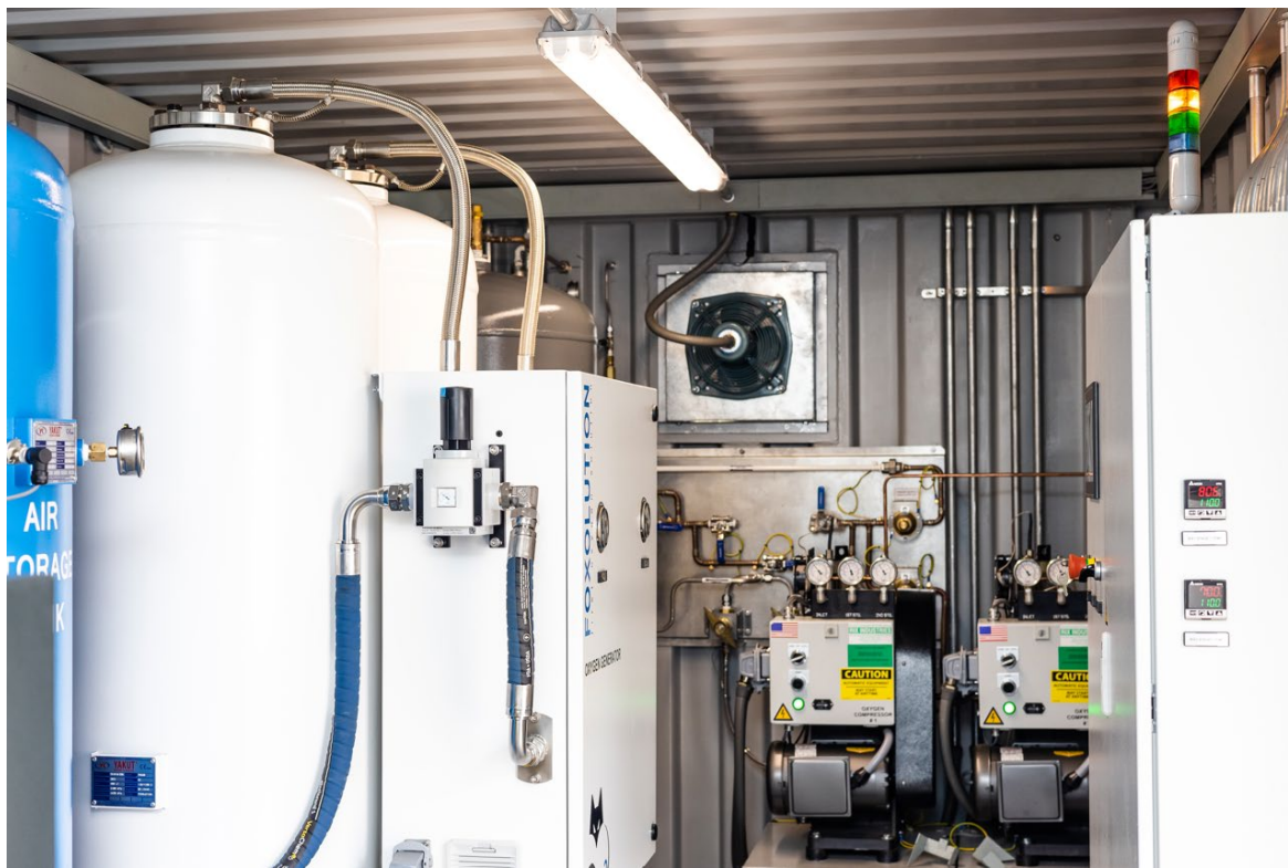
IMAGE 08: MEDFOX-185-CT-DS CONTAINERISED OXYGEN 93% CYLINDER FILLING SYSTEM INTERIOR
