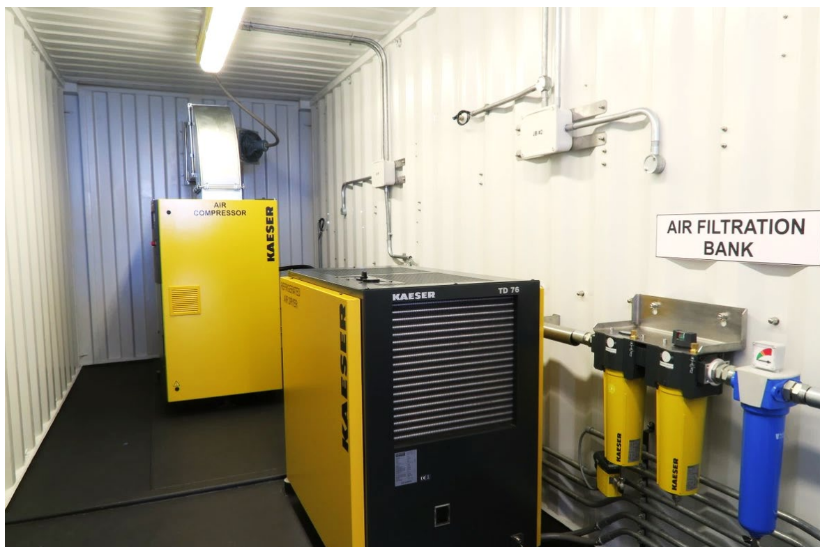
IMAGE 10: MEDFOX-300-CT-DS TYPICAL AIR SUPPLY EQUIPMENT
