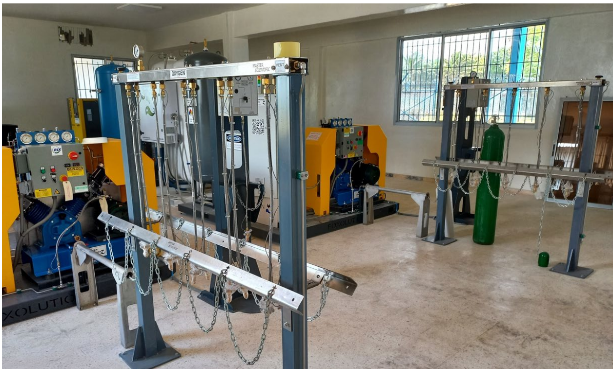
IMAGE 12: MEDFOX-300-SM FILLING MANIFOLDS AND 2V3 RIX 50 P/DAY OXYGEN CYLINDER FILLING COMPRESSORS
