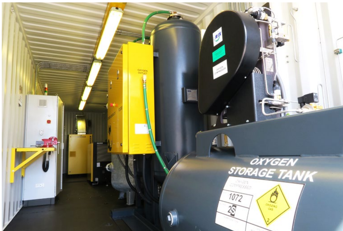
IMAGE 10: MEDFOX-300-CT-DS TYPICAL AIR SUPPLY EQUIPMENT
