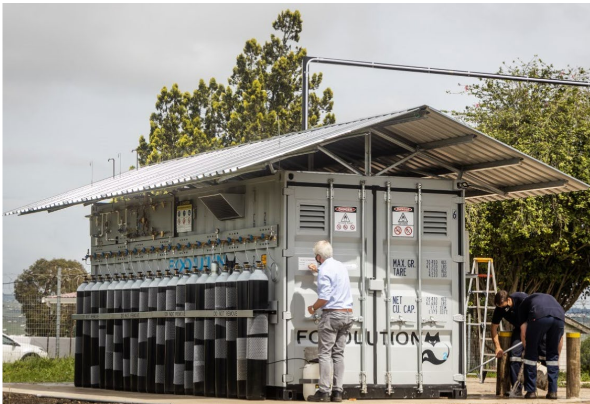
IMAGE 06: MEDFOX-185-CT-DS CONTAINERISED OXYGEN 93% CYLINDER FILLING SYSTEM EXTERIOR
